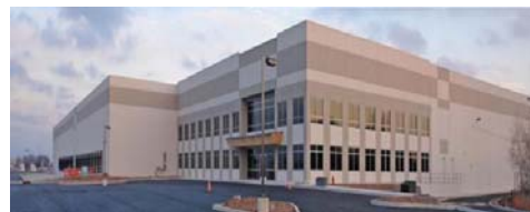
Exterior of new distribution center at New York branch of JFC International Inc.
