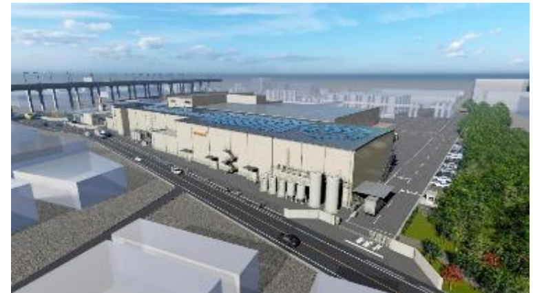
New plant of Kikkoman Food Tech Company (located in Noda City, Chiba Prefecture)
