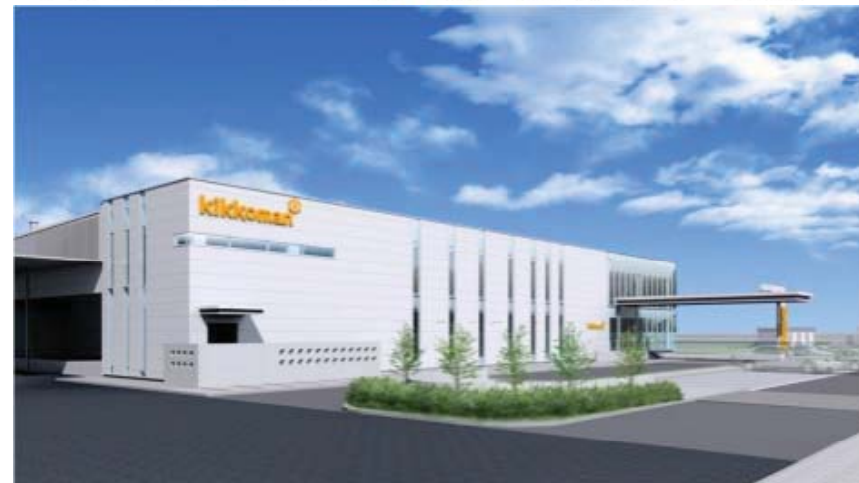
Saitama Kikkoman Company (New factory for handy Japanese-style seasoning mixes) Started production in December 2012
