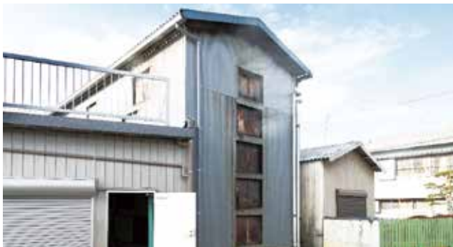
Takinaya-style baikan tower
