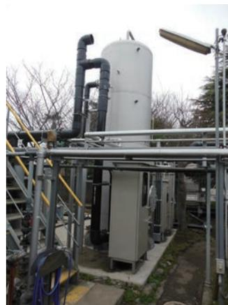
In March 2015, a pressure floatation separation apparatus was installed at the First Production Department of Noda Factory of Kikkoman Food Products Co.
