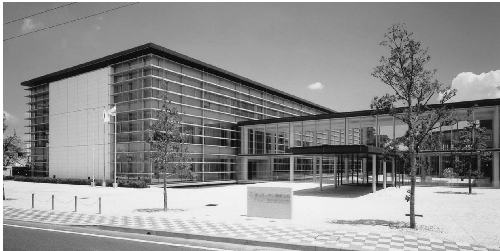
Front view of Noda Headquarters building, which harmonizes with the streets of Noda, the birthplace of Kikkoman.
