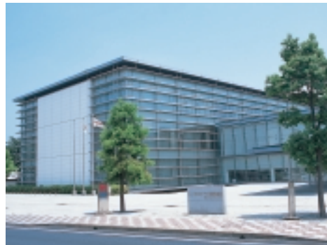
The buildings of Kikkoman's Noda headquarters harmonize nicely with the surrounding neighborhood
