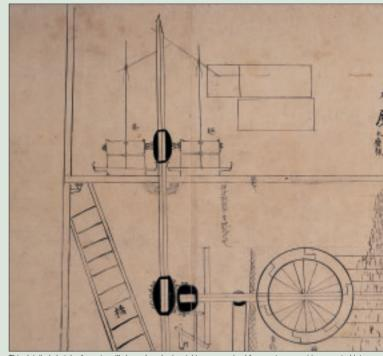
This detailed sketch of a watermill shows how horizontal torque received from water current is converted into by rotating millstones. This mechanism, which allows for two simultaneous grinding processes increased
