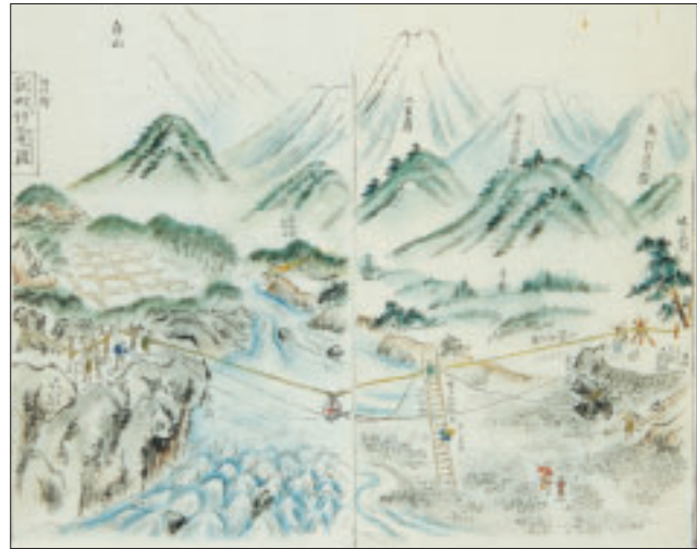
A pulley system over the river between Hatogaya and Hagimachi villages Similar systems were used at several locations throughout the Shirakawa-go district.
